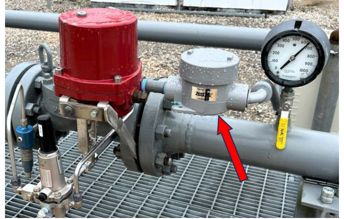
FM-4 "conduit junction box" providing the needed surge protection to ensure equipment survivability
